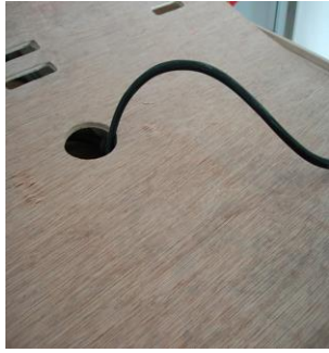
FIG-18 Pull Power Cord through Roof Cover Cover
