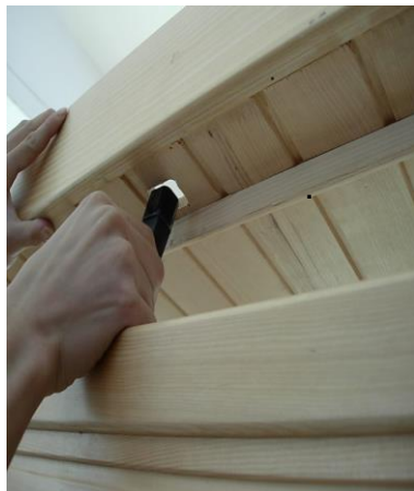
FIG-12 Slip cords/wires through corresponding holes
