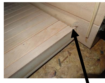
Trim molding of FRONT WALL PANEL resting on the FLOOR PANEL on the interior
