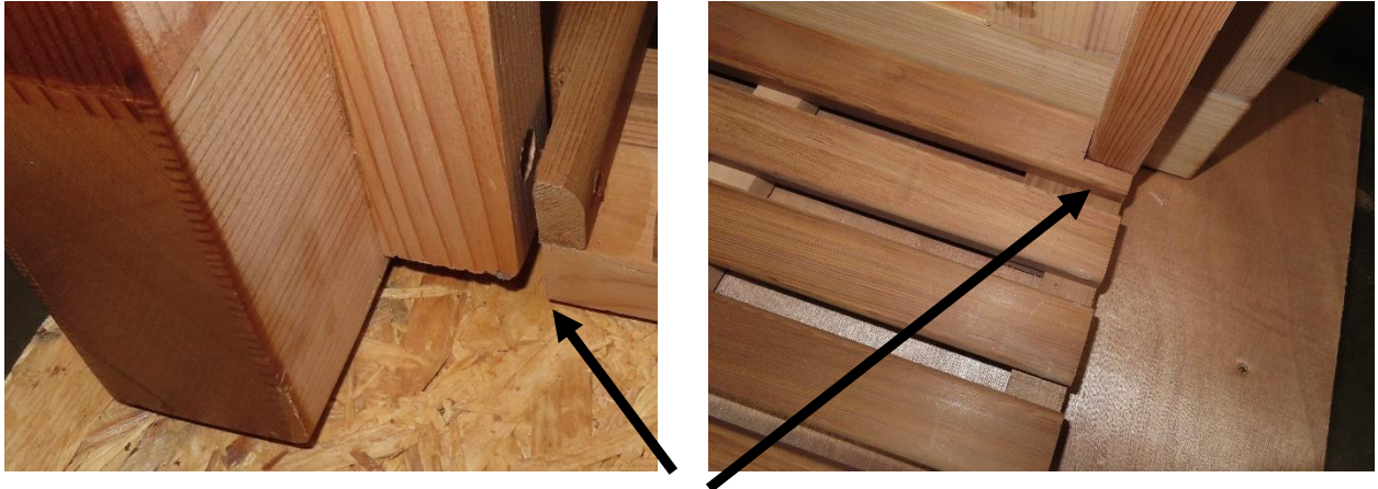
FRONT WALL fits into FLOOR WOOD LATTICE cutouts
